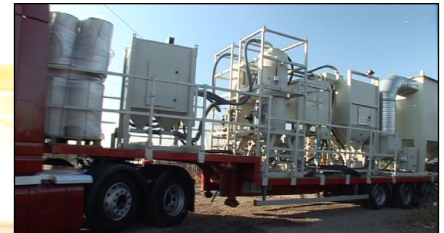
Delivery to site Walthamstow London UK February 2007
